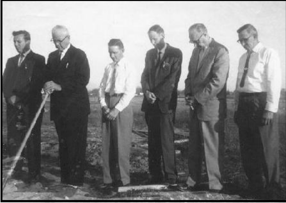
1960 Highlands MBC—Ground Breaking
